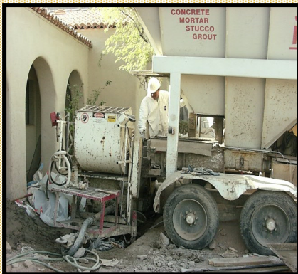
Grout being pumped under the house
