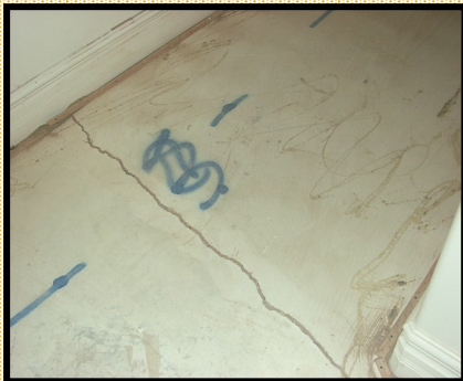
Crack in concrete slab
