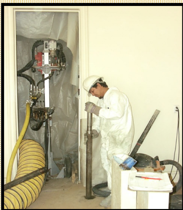
Grout being pumped under the house
